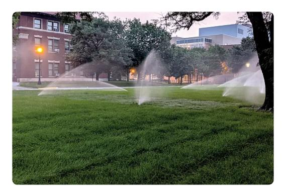
In?ground systems can reduce the environmental impact of irrigation if paired with deficit irrigation and sensors for rain, soil moisture, and evapotranspiration. Photo by Ross Braun.
