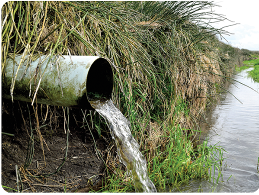
Water flows out of a tile drain into a nearby ditch. Photo by Jane Frankenberger.
